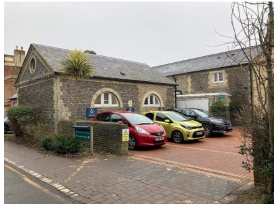
Figure 26: Examples of paving treatments in Goring Hall grounds.
