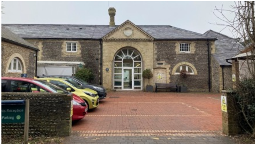
Figure 21: Former stable building at Goring Hall
